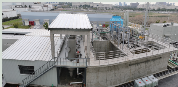
Figure: Wastewater treatment station
