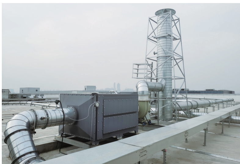
Figure: Exhaust gas disposal center
