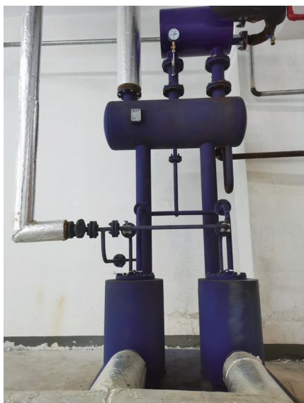
Figure: Condensate water recovery system
