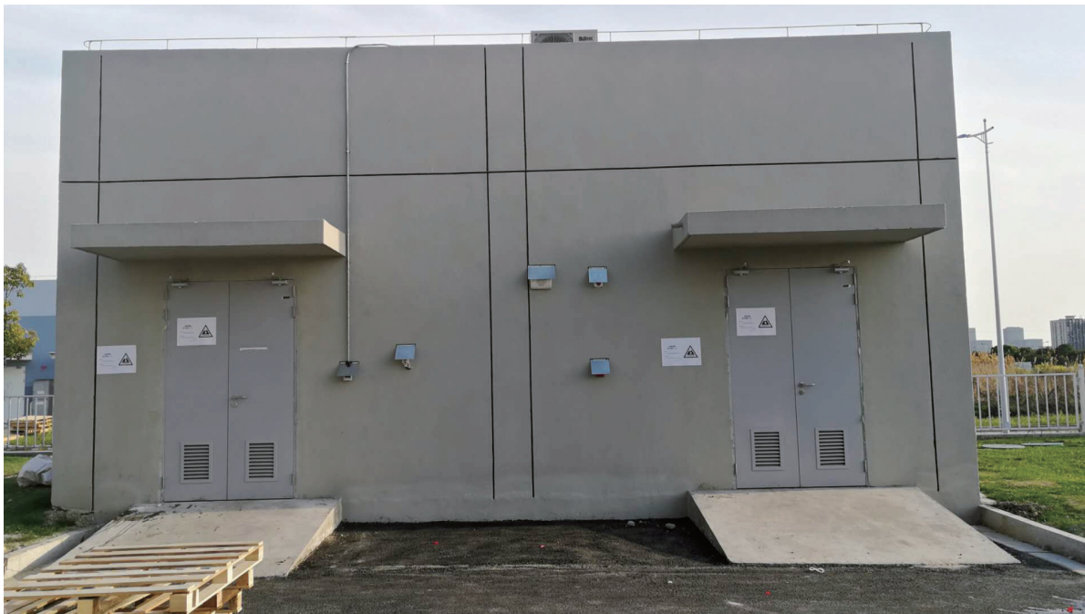
Figure: Hazardous waste warehouse
